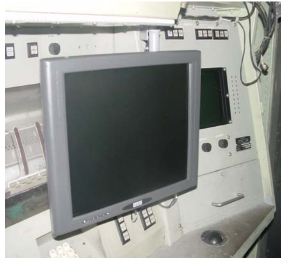
DMK Display Installation
